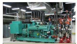
**Application:** Emergency standby system including two DQGAA (1250 kWe) and one DQGAB (1500 kWe) provided by Cummins.
