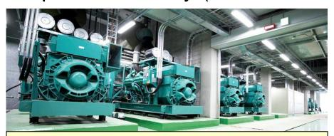
**Application:** Standby power system including seven C2000 D6 (2000 kWe) generator sets provided by Cummins.
